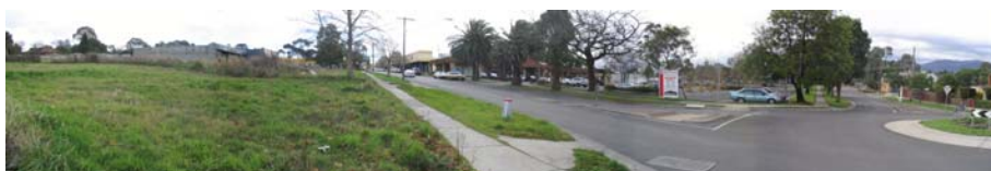
Above: There is significant potential in and around the retail core for new housing above retail and office developments (e.g. corner of High St and Pine Road).
