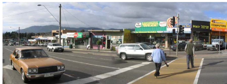
Above: Many existing shop frontages present poorly to the street with little consistency in signage, verandahs or colours.
