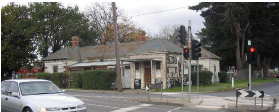
Above: The Bayswater Wine Café is on a prominent site on the edge of the activity centre. With renovation and investment, this could become a landmark building.
