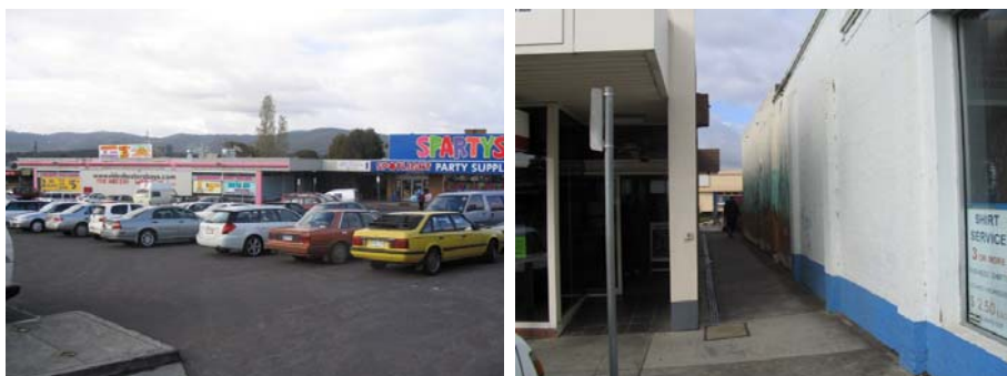
Above: Car parking in front of shops provides a poor interface with the street. Narrow pedestrian access way with little potential for passive surveillance creates an inhospitable environment for pedestrians at night.
