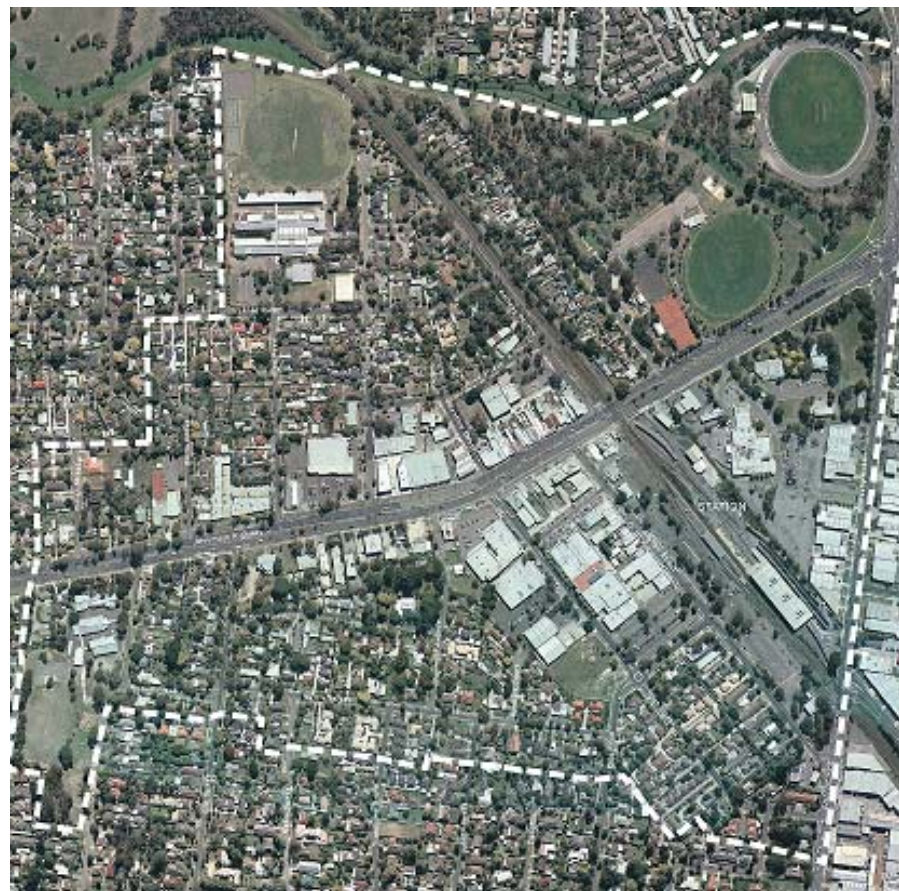
Aerial photograph (2003) showing Bayswater Activity Centre and the study area
