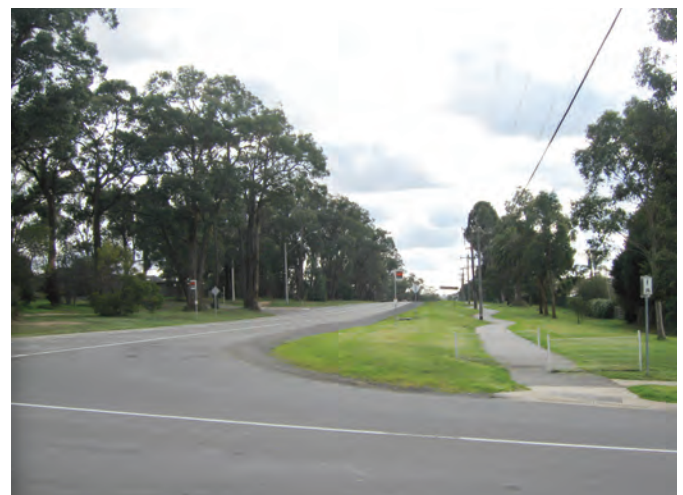
Mountain Highway, The Basin with an off-road shared path
