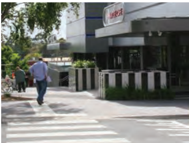
Mountain High Centre, Bayswater showing distinct planters at the entrance
