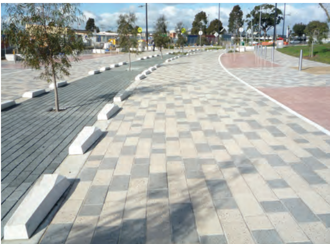
Shared street, Main Street, Broadmeadows, showing various materials to decrease driver speed
