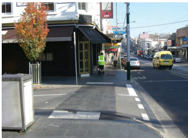
Crossing point, South Yarra showing the road raised to pedestrian level and paved in the foot path material, to prioritise pedestrians
