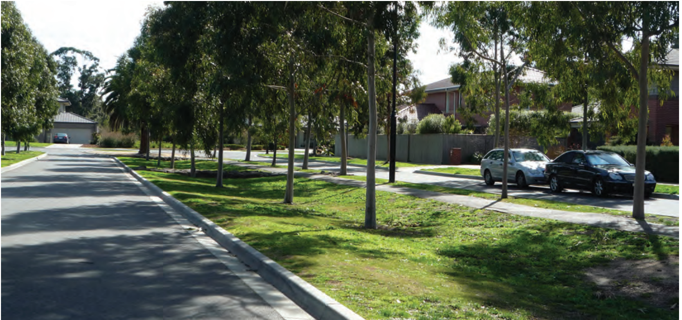
A street with a central swale to capture and clean the storm water from the carriageway, Springthorpe, Macleod
