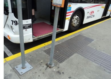
Footpath at same height as bus entrance and edge of footpath clearly visible
