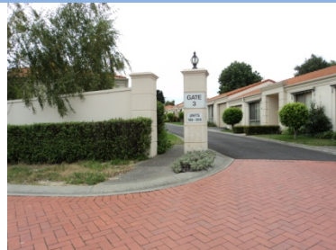
Pedestrian gate much narrower than vehicular gate
