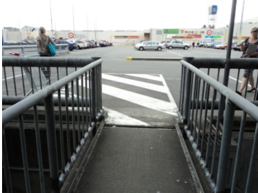
Footpath leads directly into car park!
