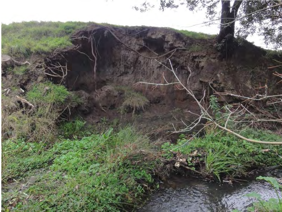
Figure 7. A dangerously undercut bank.
