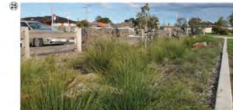
Provide a new vegetated drainage swale to capture and treat stormwater runoff along the eastern edge of the new multipurpose courts and youth/ community facilities.
