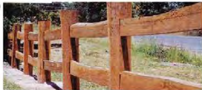
Remove existing 1.8m high chain wire mesh fence along Simon Ave and replace with a timber post and rail fence.
