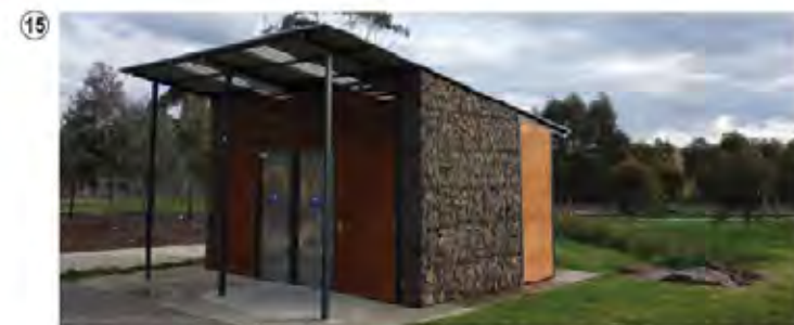
Remove existing degraded public toilet facility within the playspace. Provide new public toilet facility in a more accessible location between the playspace and new multipurpose courts and youth/ community facilities.
