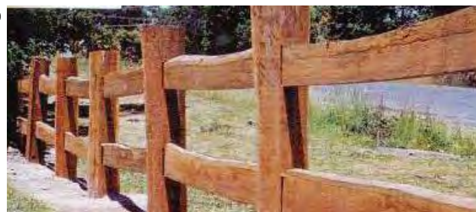
Remove existing 1.8m high chain wire mesh fence along Simon Ave and replace with a timber post and rail fence to improve site permeability.
