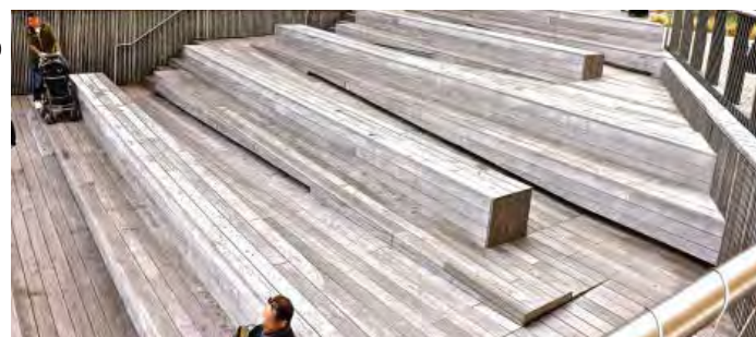
Provide a new DDA compliant access link between the playspace and proposed multiplay courts and youth/community recreational facilities. Incorporate terraced seating overlooking the open grassed area for amenity and event usage.
