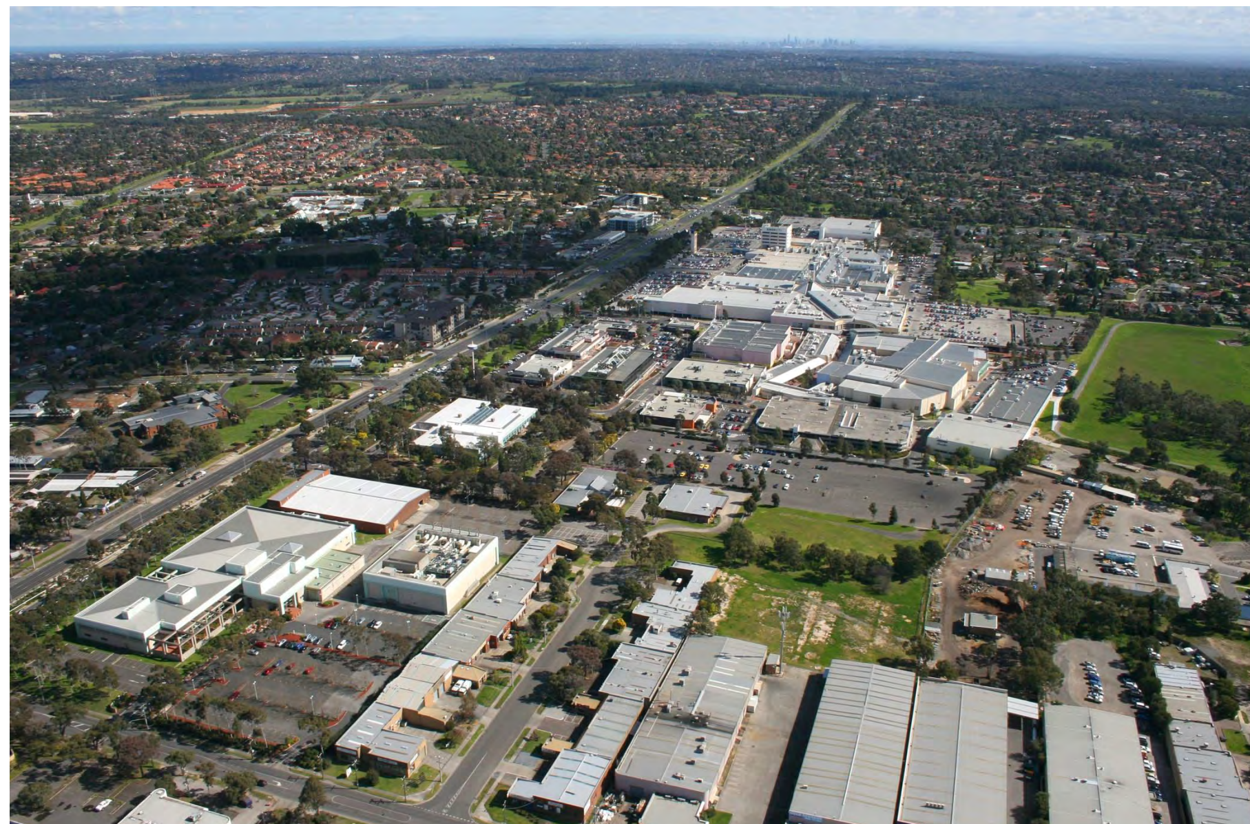
Figure 11 Aerial photo showing Knox Central's built form
