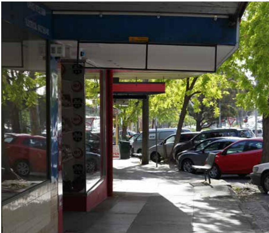
Generally continuous weather protection provided along Burwood Highway, east of Dawson Street.
