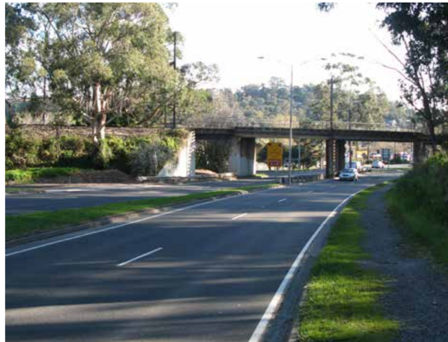
Railway bridge that define entry in the Activity Centre from the east
