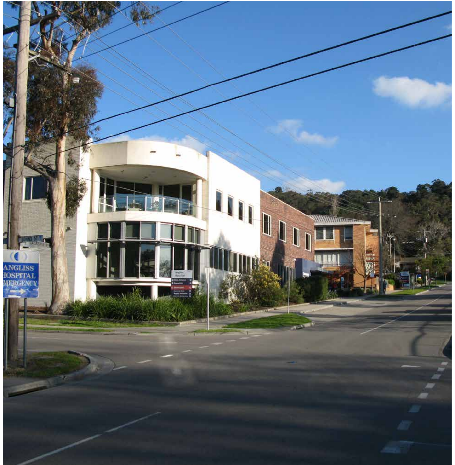
The Angliss Hospital, located along Talaskia Road
