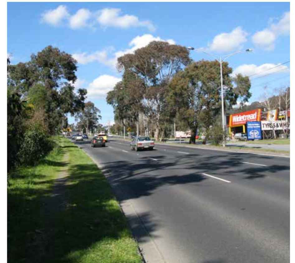
Burwood Highway, west of Glenfern Road, travelling west towards Upper Ferntree Gully
