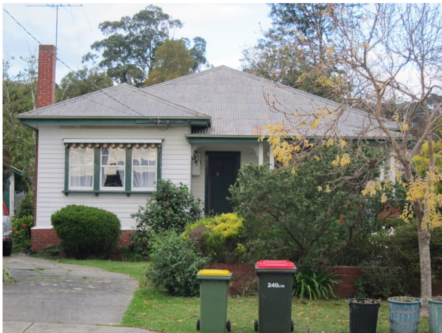
Figure 13 House, 3 Rollings Road, Upper Ferntree Gully (Source: Context 2015)
