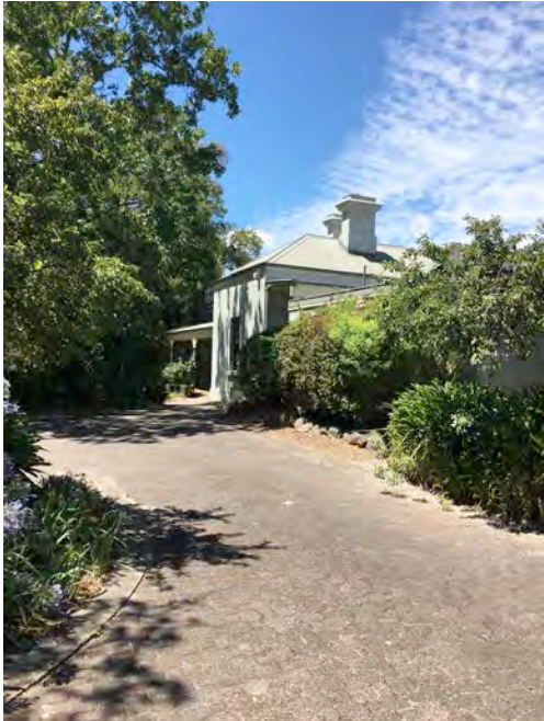
Typical driveway pathway paving throughout site, presumably installed in the 1980s
