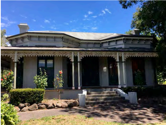
View of the front of the homestead. Note French doors and roof profile, steps and rocks to garden bed
