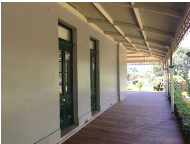
View of verandah (Note: recent verandah floor)
