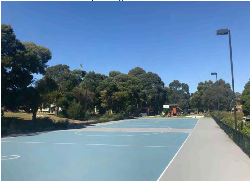
The reserve is home to three lit acrylic-surface hard courts in good condition that are only line-marked for netball.
