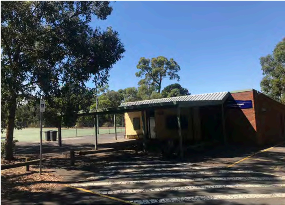
The existing pavilion and courts (to be demolished).
