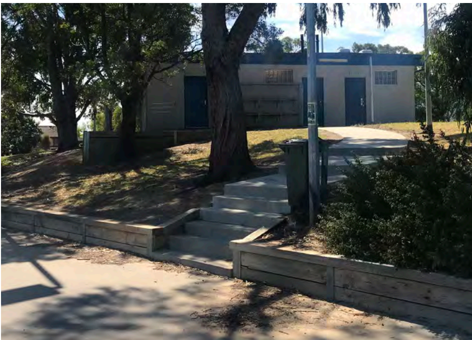
Steps and path leading to toilet/chamnge facilities, located within the football/ cricket pavilion.
