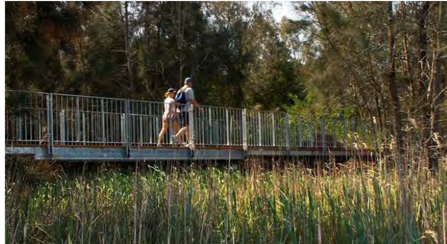
Bridge over sensitive vegetation
