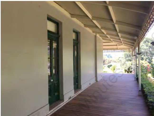
View of verandah (Note: recent verandah floor)
