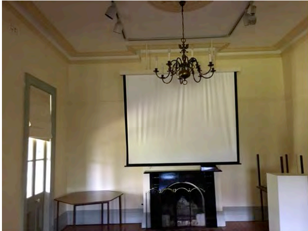
View of room on left of hall showing original fireplace and typical cornice, skirting and architrave detail
