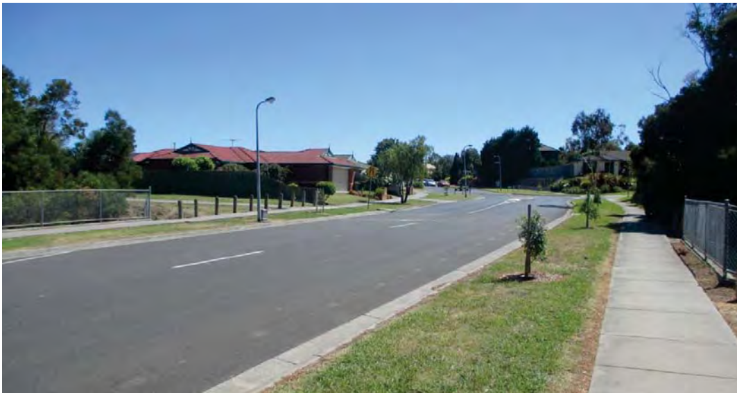
Figure 3 Typical road asset under Council's responsibility
