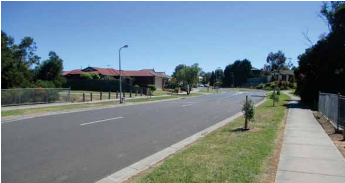
Figure 3 Typical road asset under Council's responsibility
