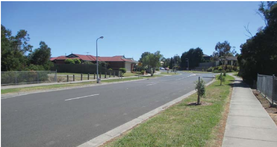
Figure 3 Typical road asset under Council's responsibility
