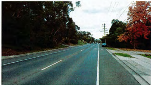
Figure 2.8: Forrest Road (Looking West)
