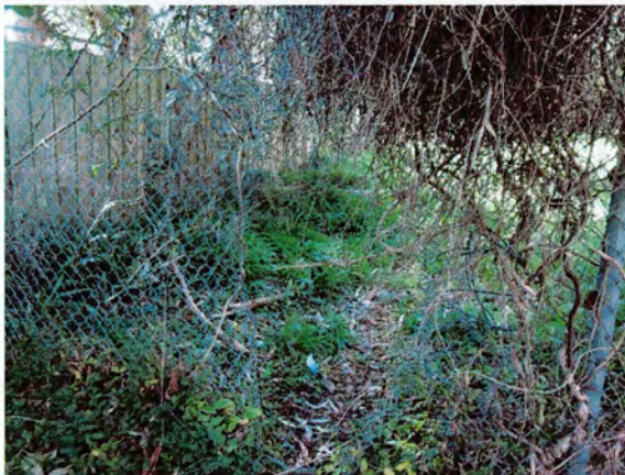
Photograph 5: Fence in disrepair
