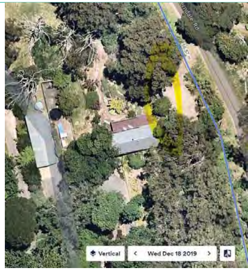
2019 – retaining wall possibly in same location
