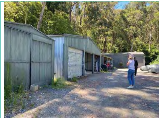
Site inspection photo of said sheds
