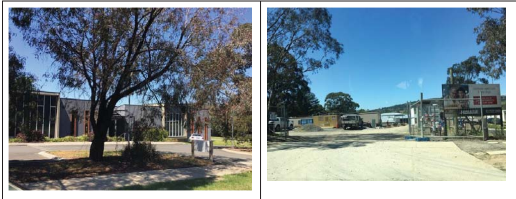
Figure 8 Le John Street: The Rowville Baptist Church and a residential aged care facility (under construction in October 2019)
