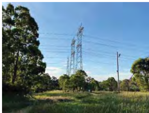
Figure 10 - Adjacent high-voltage overhead wires adjacent to site
