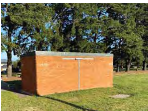
Figure 5 - Existing public amenities block
