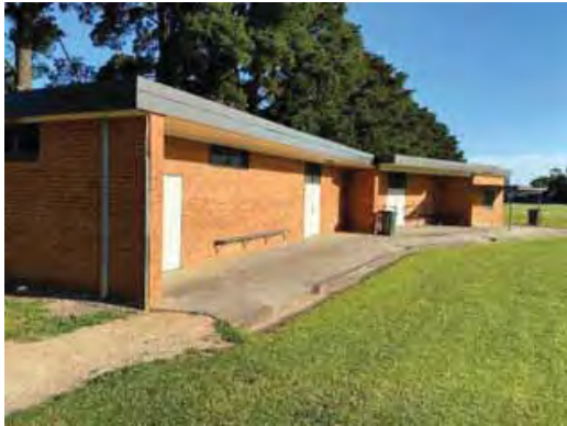
Figure 1 - Existing changeroom / pavilion
