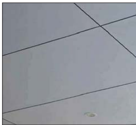
FC-1 Expressed Joint Sheet Cladding Soffit
