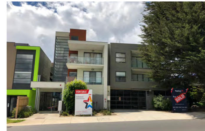
Example of recent development with a ground level vehicle interface.
