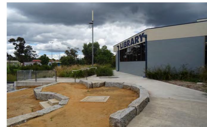
Recent public realm works at Boronia Park.
