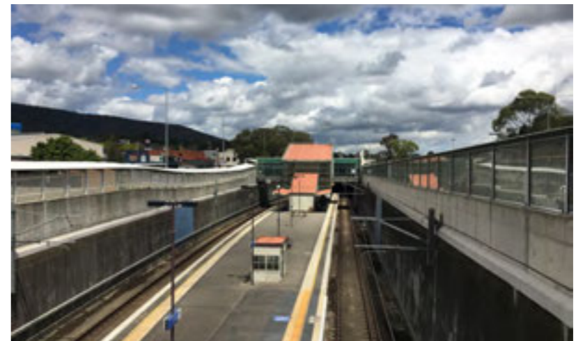
The grade separated Boronia Railway Station
