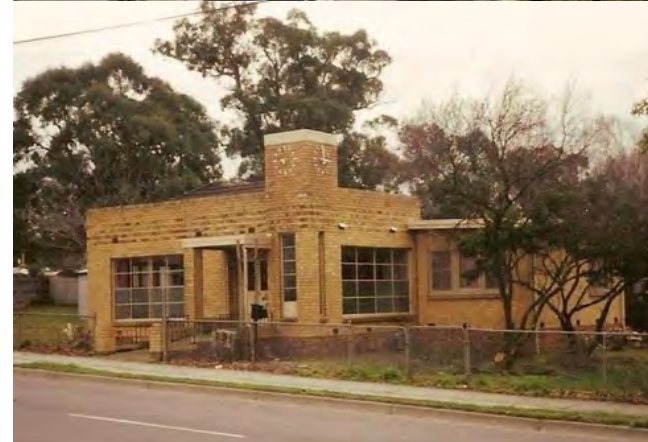
Looking west to 765 Mountain Highway recommended for further assessment of inclusion in the Heritage Overlay, from the raised road deck/pedestrian ramp of Mountain Highway at the corner of King Street. Historic image prior to overpainting (from https://www.facebook.com/Bayswater-History-and-Community-News-561695913882255/photos/4452124838172657 )
