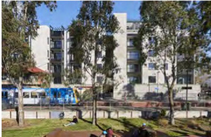
Nightingale 2.0 adjacent to Fairfield Station is an excellent example of previous Vic Track land used for residential development.
