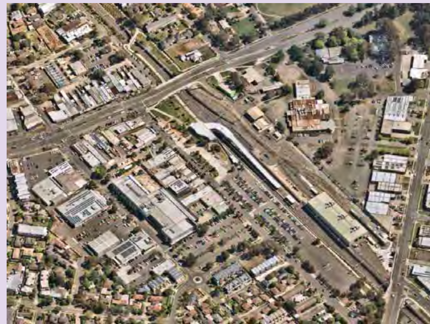
Bayswater Railway Station and Environs in 2021
