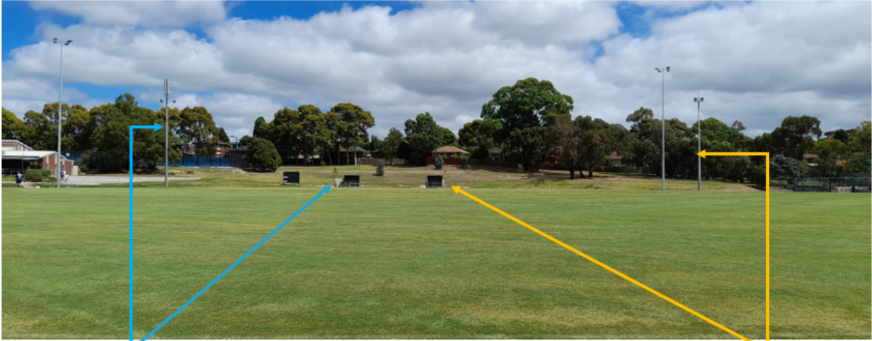
Figure 1 – Existing mobile phone base stations at Templeton Reserve
