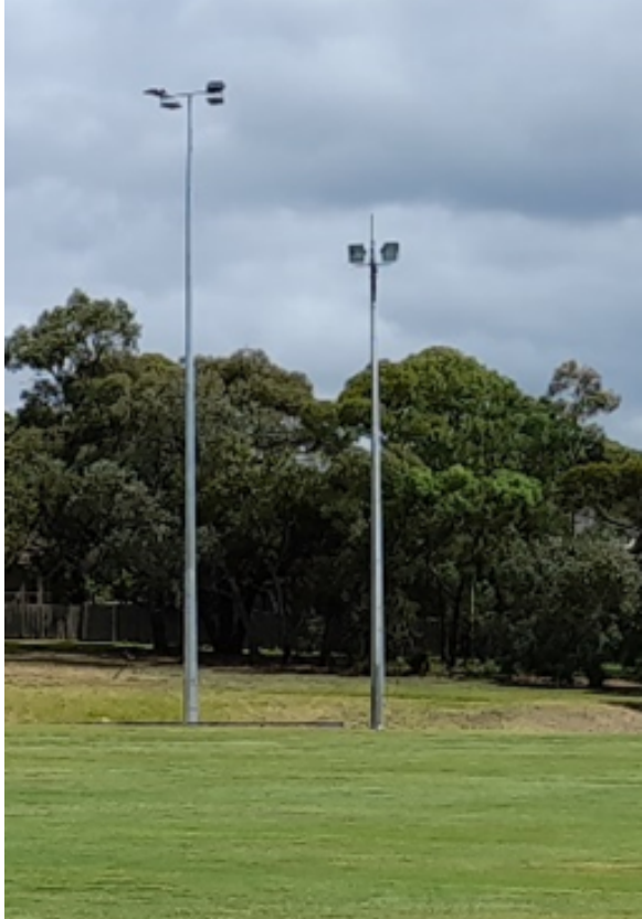
Figure 8 – Existing 25m floodlight tower and 18m Telstra telecommunications pole
