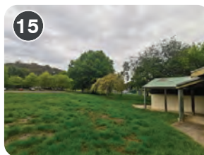
15 Existing athletics clubhouse - outdated and disjointed from the high jump area
