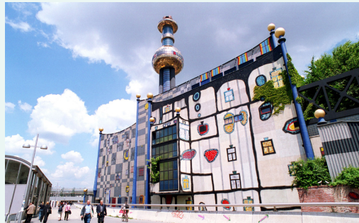
Spittelau Waste to Energy Facility, Austria
