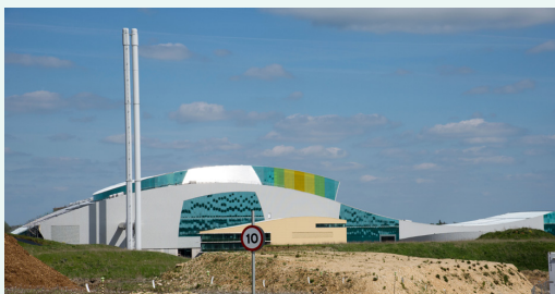
Ardley Energy Recovery Facility, UK
