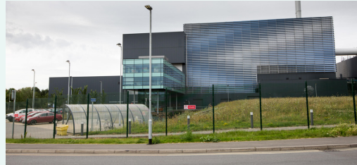
Suffolk Energy From Waste Facility, UK
