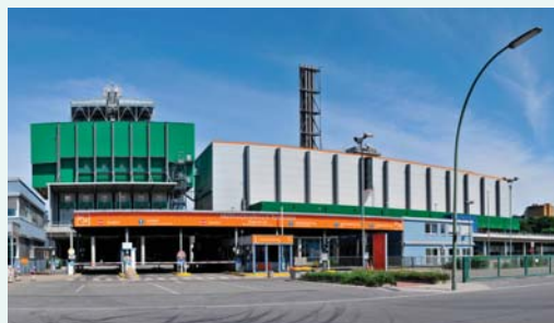
Ruhleben Waste to Energy Facility, Germany
