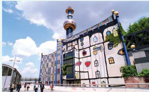
Spittelau Waste to Energy Facility, Austria
