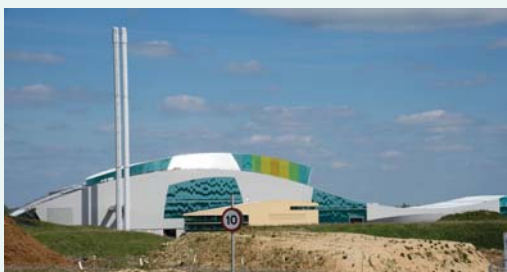
Ardley Energy Recovery Facility, UK
