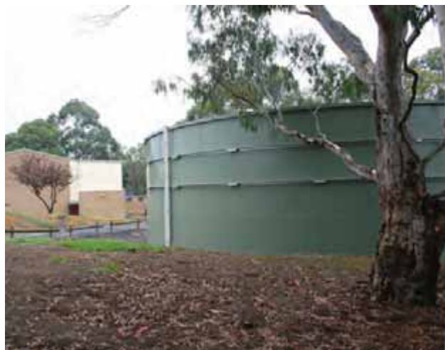
Bayswater Oval Siemens water recycling
