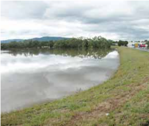
Lewis Park retarding basin, holding water
