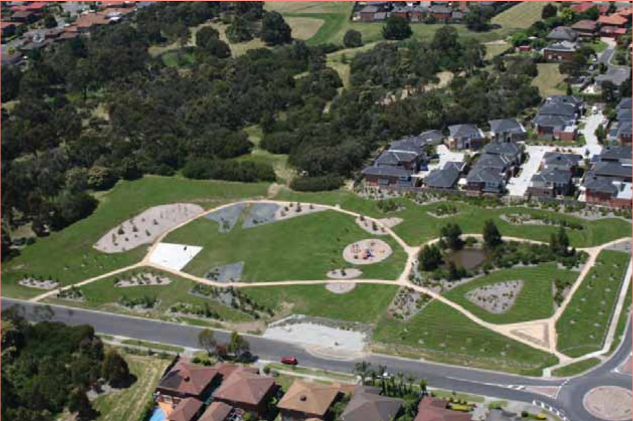
Aerial photograph of Jenola Park, Wantirna South
