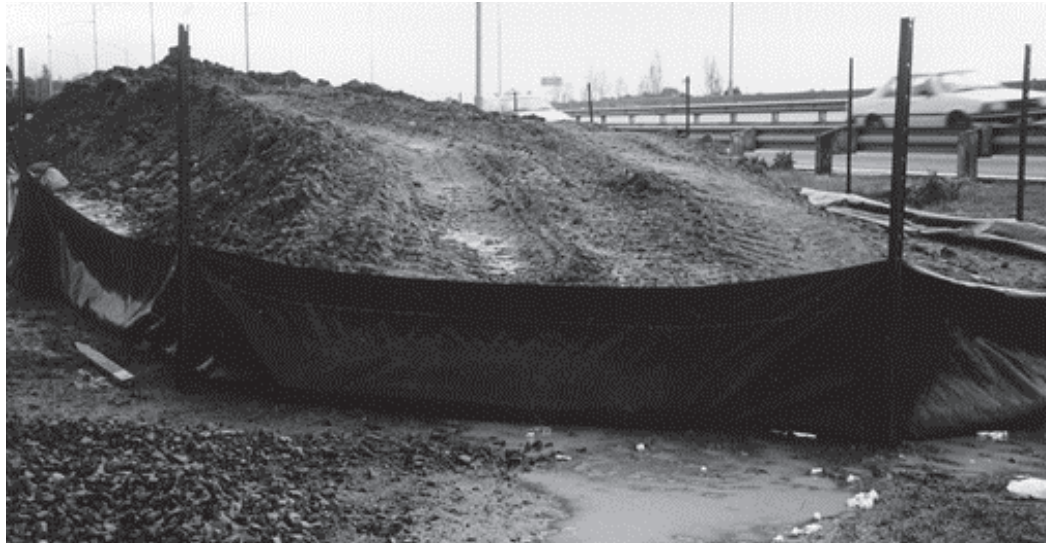
Figure 6.13 A silt fence around a stockpile.
