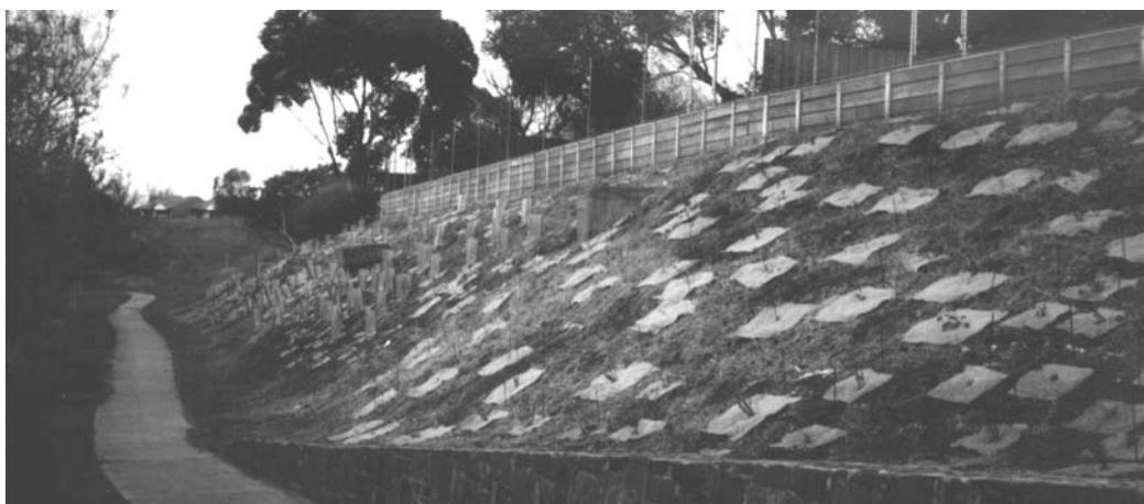
Figure 6.10 Stabilisation and revegetation protect soils from erosion.
