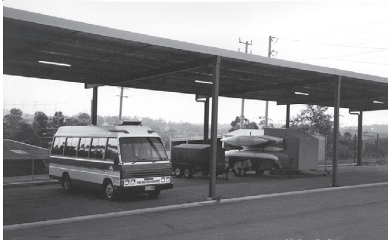
Figure 6.2 A temporary storage facility, undercover and with a spoon drain to redirect surface flow (City of Manningham).
