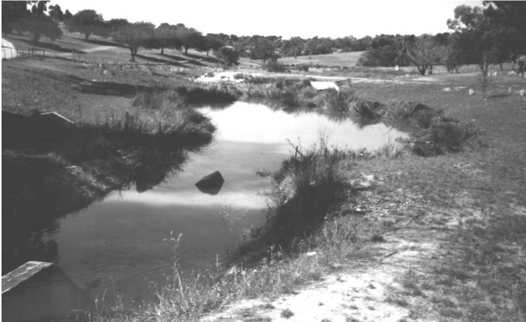
Figure 7.33 Inlet zone providing coarse sediment capture, Ruffeys Creek, Doncaster.
