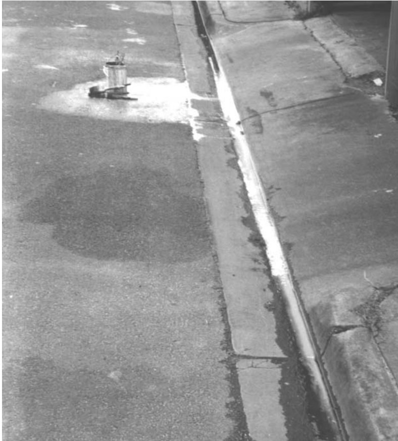
Figure 6.5 Many building maintenance practices can pollute stormwater.
