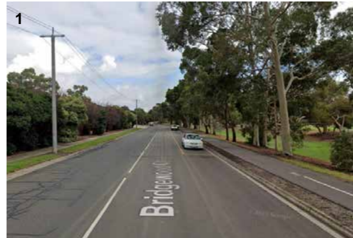
1 Bridgewood Court / Blind Creek Existing road to be reconsidered to accommodate a direct built form interface to Blind Creek / Lewis Park
