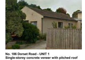
No. 186 Dorset Road - UNIT 1 Single-storey concrete veneer with pitched roof
