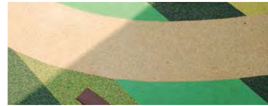
3 WETPOUR RUBBER IN VARIOUS COLOURS - ACCESSIBLE PATHS THROUGH PLAYGROUND
