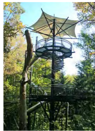
VIEWING TOWER - STEEL STRUCTURE WITH ACCESSIBLE PLATFORM (NOM. 1.5M OFF GROUND) AND STAIRWAY TO HIGH VIEWING PLATFORM (6.5M OFF GROUND) WITH CANOPY OVER. ALLOW FOR SECURITY PROVISIONS
