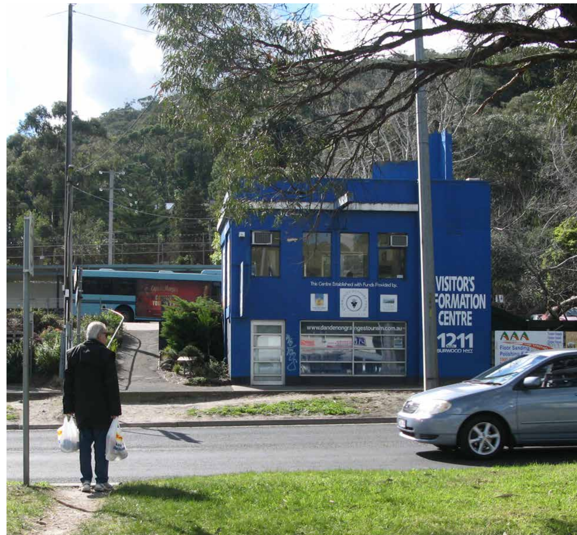
The Visitors Information Centre is managed by Yarra Ranges Tourism and the building is valued by the local community
