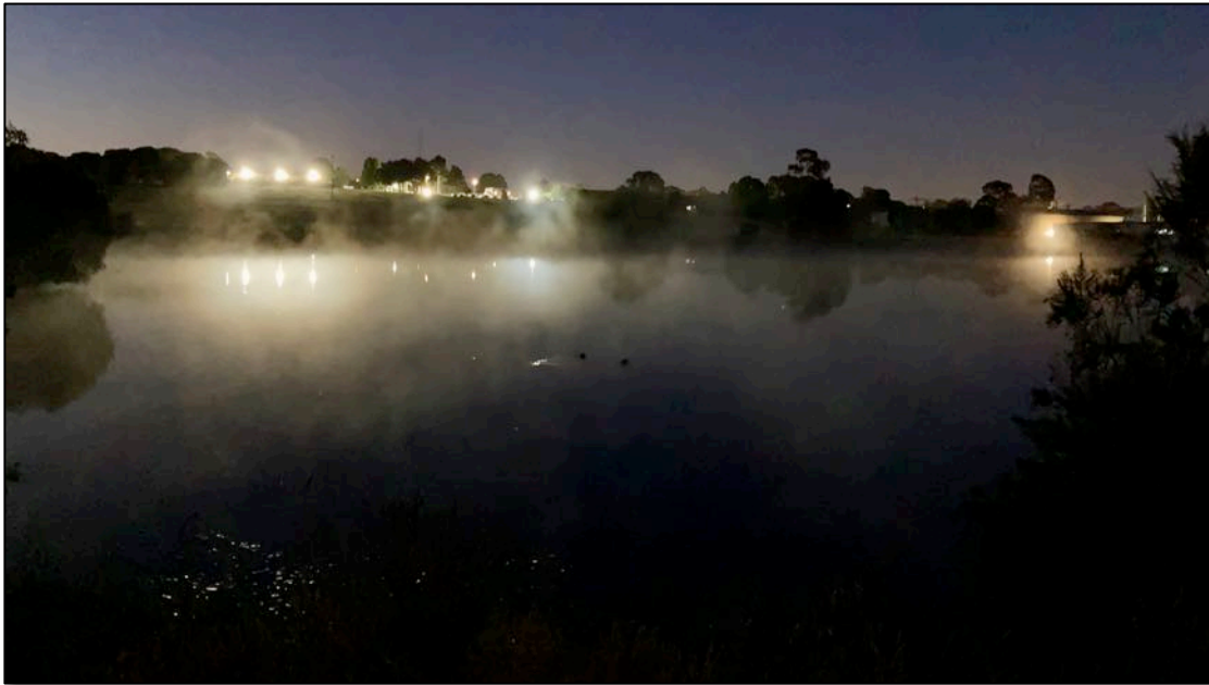
Pre-dawn looking south across the dam
