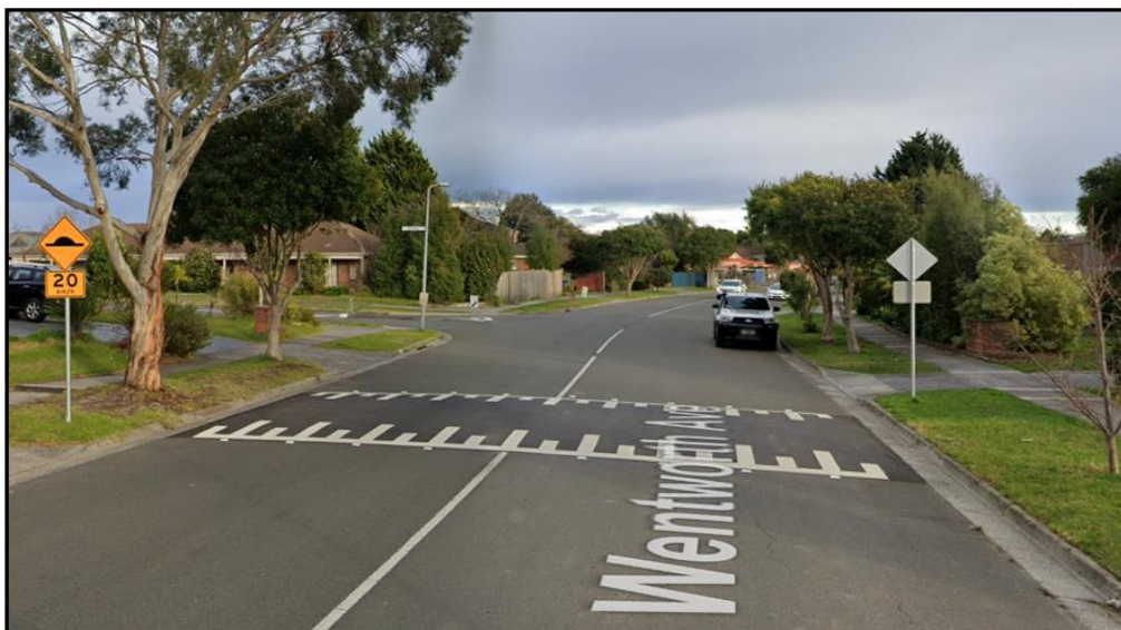
Example of speed hump on local road.
