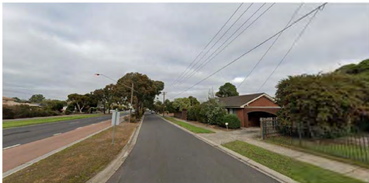
V2: VIEW LOOKING SOUTH FROM STUD ROAD SERVICE LANE
