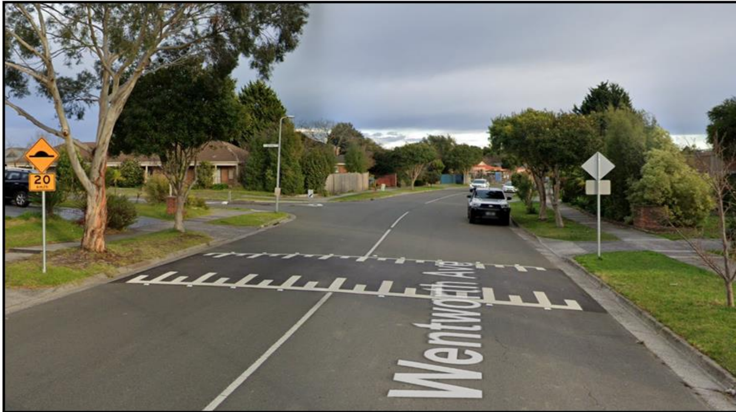
Example of speed hump on local road.
