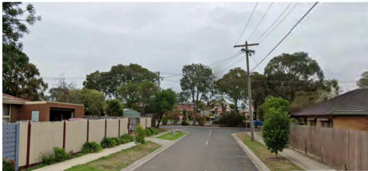
V1: VIEW OF EXISTING SITE CONDITION ALONG MICHELE DRIVE
