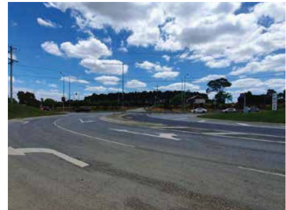
View 8 - High Street Road intersection from George Street.
