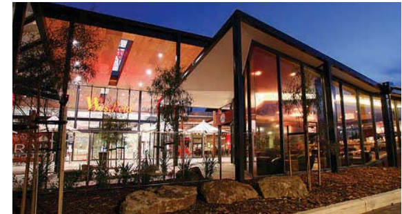
Address adjoining footpaths, car parks and public spaces with active and permeable facades.
