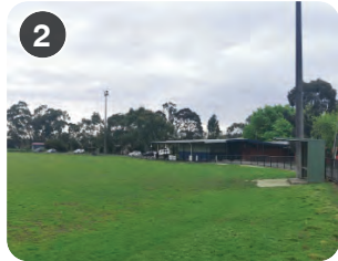
2 Oval 1 pavilion is disjointed from oval 2 and cricket nets- opportunity to consolidate uses
