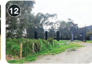
12 Cricket nets area- lack of DDA access and lack of gathering space
