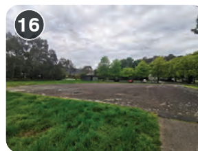
16 Former netball courts in poor condition, currently used as high jump area - possible new playspace / intergenerational space location
