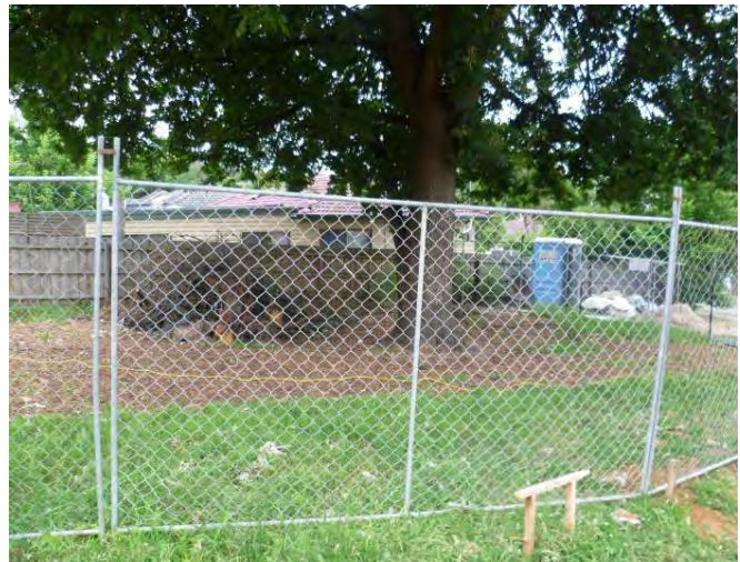
Tree Protection Fence with suitable fencing
