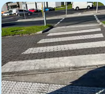
TGSI does not align with safe travel direction and is same colour as path surface. WM
