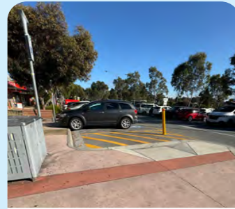
Share zone adjacent to accessible car park which is connected to the footpath and protected by a visible bollard. WM
