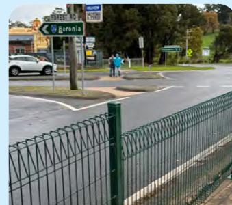
No TGSI in pedestrian refuges. TBT
