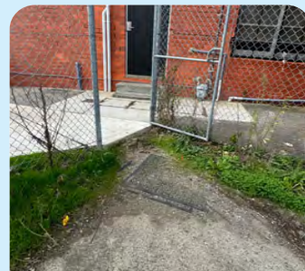
Step at end of footpath through gate difficult for PMDs to use. SV
