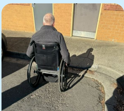
Bullnose edges difficult to navigate. KF
