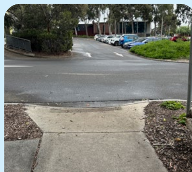
Footpath leads into roadway and does not connect with another footpath. RCC
