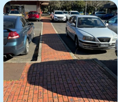
Footpath too narrow, difficult for carer to walk alongside person using wheelchair. FTG
