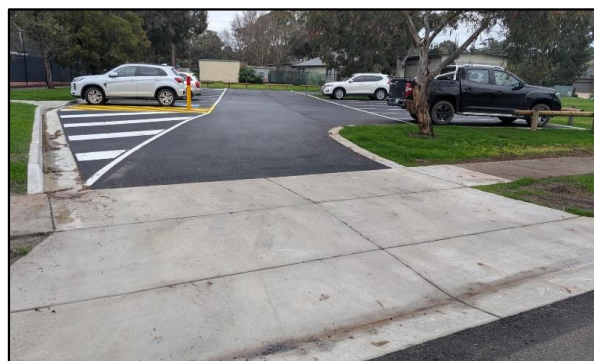
Carpark upgrade in Wantirna South to service Knox City Tennis Club and Orana Neighbourhood House.
