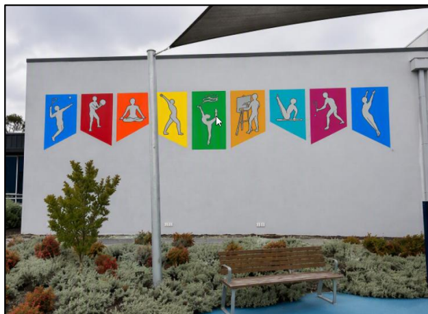
Building artwork restoration at Carrington Park Leisure Centre in Knoxfield.
