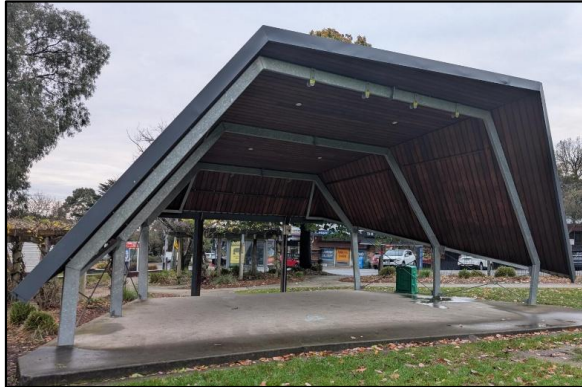
Various improvements at The Basin Triangle Reserve in The Basin, including soundproofing the stage shelter.
