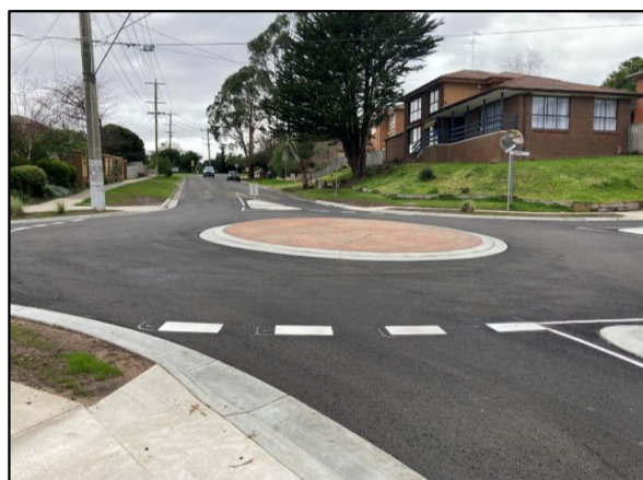
$10.6 million invested in roads (e.g. Blackwood Park Road reconstruction in Ferntree Gully).
