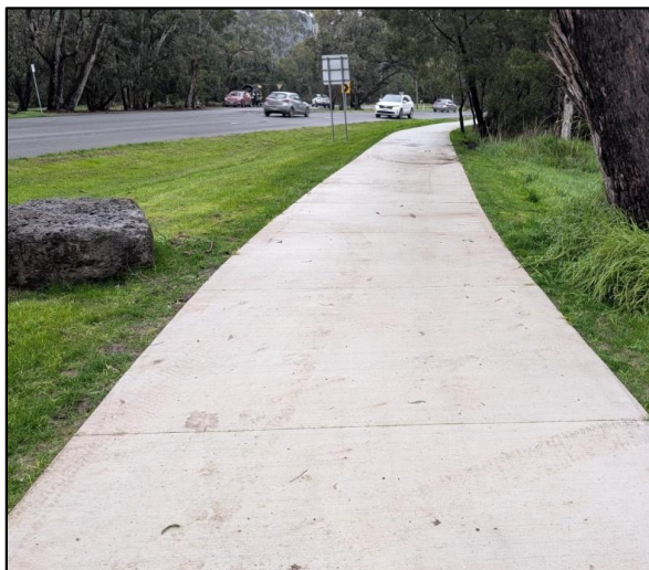
Stage 1 of a new shared path along Liverpool Road in The Basin.
