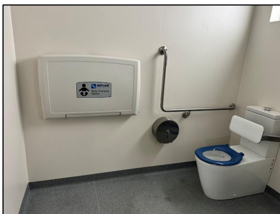
New accessible toilet at H.V. Jones Reserve Community Hall in Ferntree Gully.
