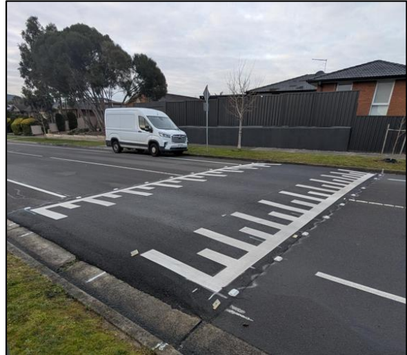
Local Area Traffic Management on Eildon Parade in Rowville, seeing the installation of seven speed humps.
