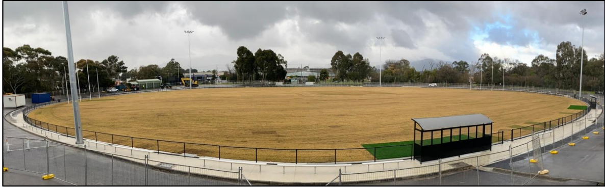
Major sportsfield renewal of Marie Wallace Bayswater Oval in Bayswater, Knox's premier football and cricket facility.
