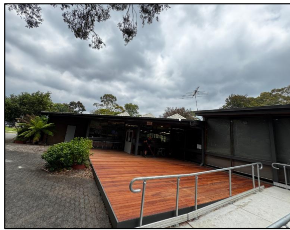
Decking improvements at Ferntree Gully Community Arts Centre & Library in Ferntree Gully.
