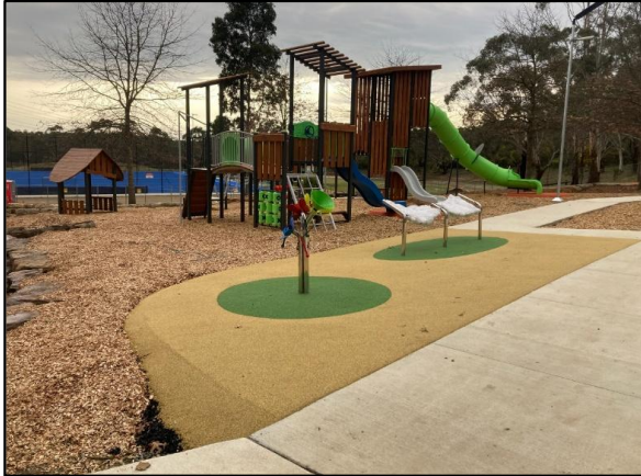
New playspace at Wantirna Reserve, Wantirna, as part of various Masterplan Implementation initiatives delivered.
